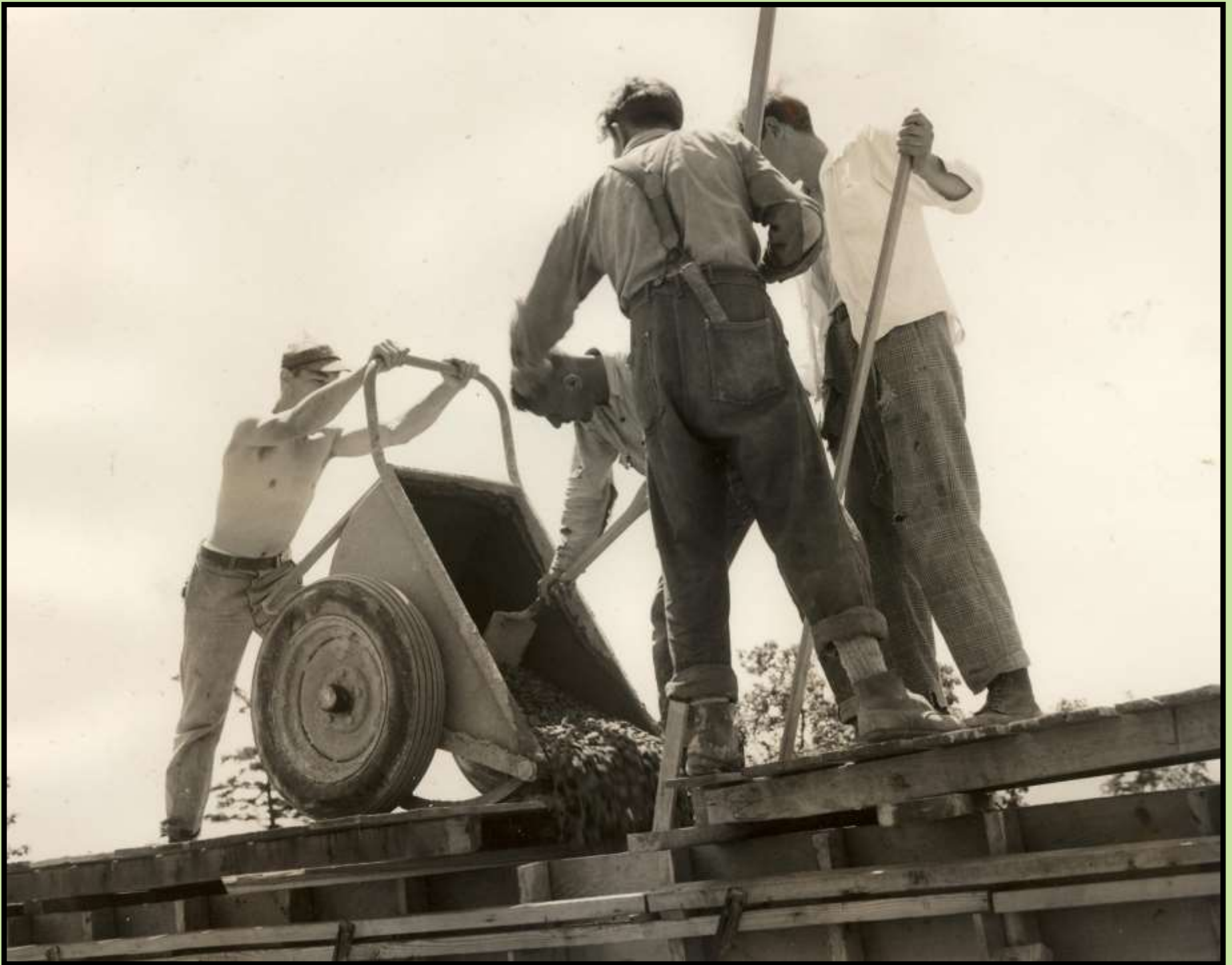
Construction of Rithet Reservoir, 1949 (1983-008-001b)
