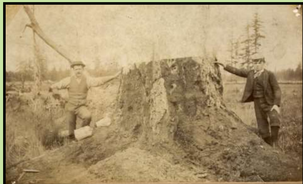
G. McMorrان Sr. & R. Maynard's grandson blasting stumps, 1895 (1989-008-196)
